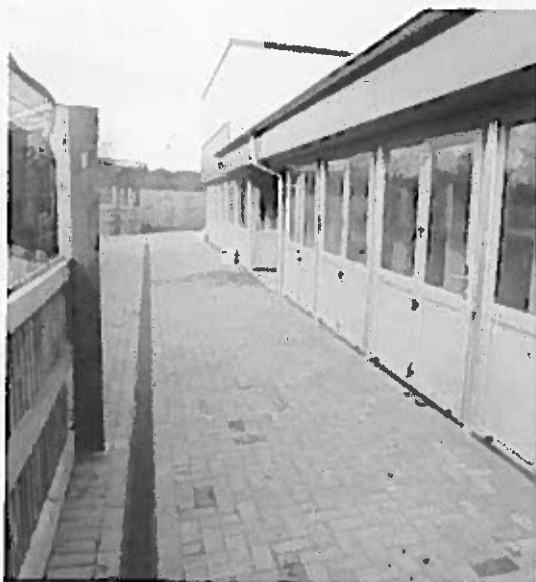
Safe area outside kennels and hard surfacing
