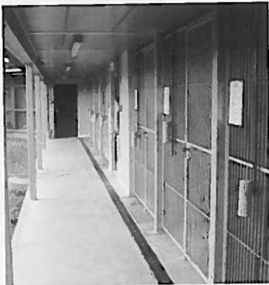
Protected external runs (showing drainage)
